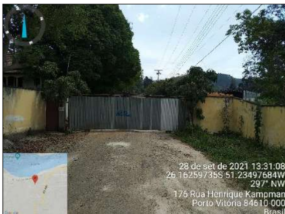
Entrada principal do complexo industrial
